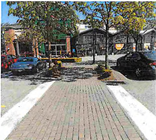
Figure 58: Curb extension and raised crosswalk
