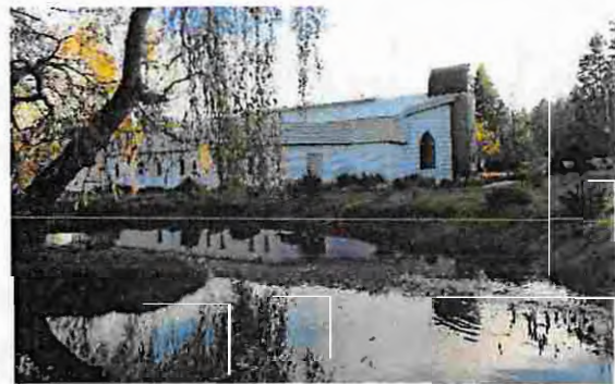
Figure 25: St. Philips by the Sea Anglican Church, in Lantzville
