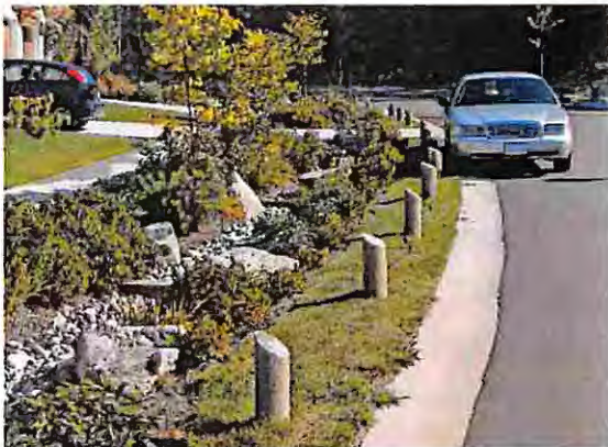
Figure 35: Storm water source controls – infiltration swale
