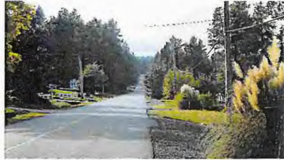
Figure 21: Roads in Lantzville are built to a rural standard, without curb and gutter or sidewalks
