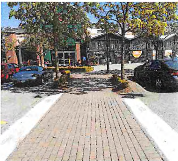
Figure 58: Curb extension and raised crosswalk
