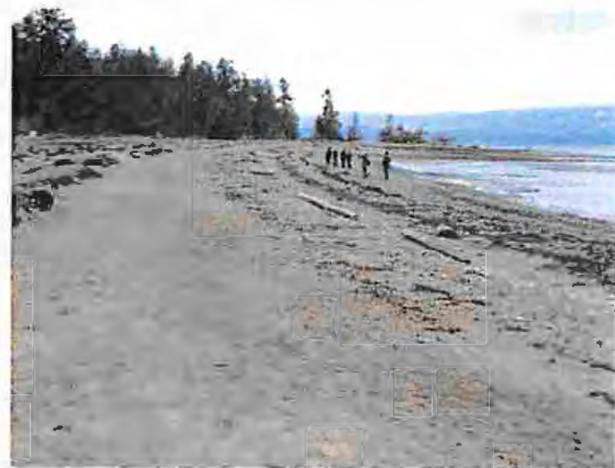
Figure 80: At Rathtrevor Provincial Park, a seawall causing waterfront erosion was replaced by beach nourishment sands and gravels in a "Green Shores" approach
