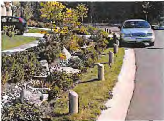
Figure 35: Storm water source controls – infiltration swale
