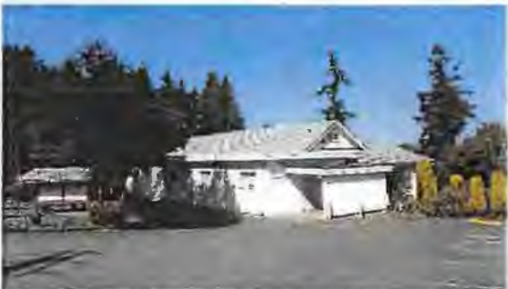
Figure 16: Costin Hall is Lantzville's primary community gathering space, but is also an aging building that will require renewal or replacement in the future
