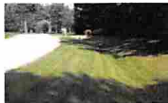
Grass stormwater swale along roadway
