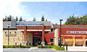
Example of a larger-scale 2-storey progressive care facility - Campus of Care in Nanaimo
