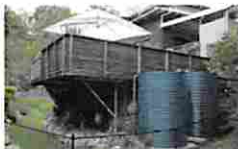
Rainwater capture tanks on a single-family home
