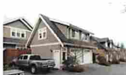
Carriage Home over a laneway garage
