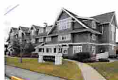
3- Storey Seniors Care Facility - Qualicum Manor, Qualicum Beach
