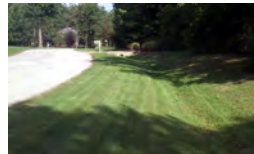
Grass stormwater swale along roadway
